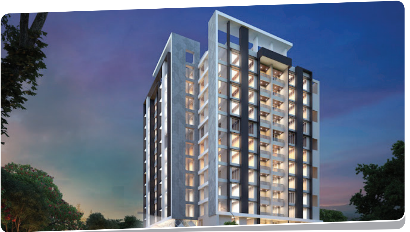
Life Style Properties Bhubaneswar | Developers : Life Style Properties Pvt. Ltd B+G+12 | Area : 2,00,000 Sqft
