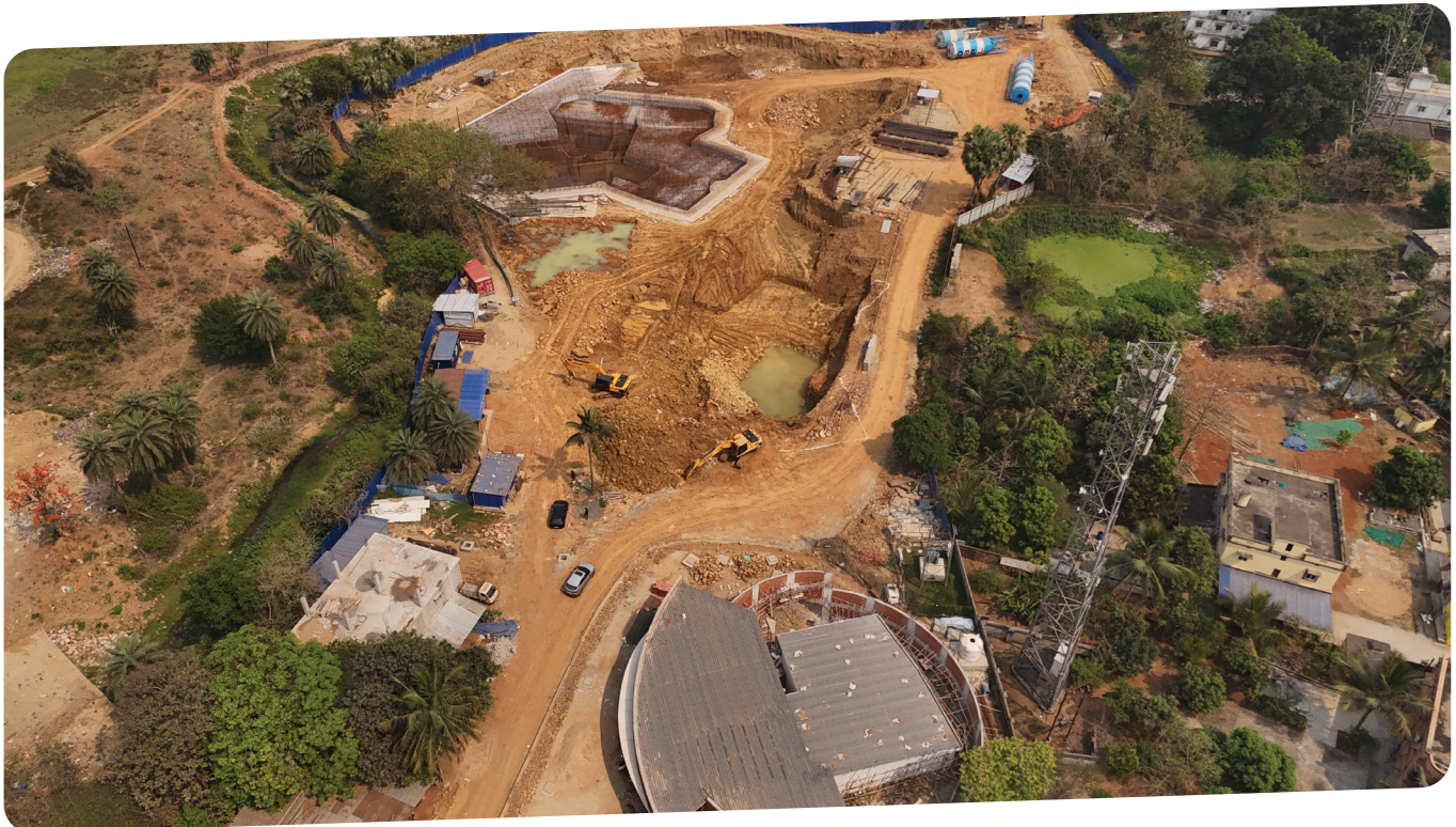
Current stage of Construction
