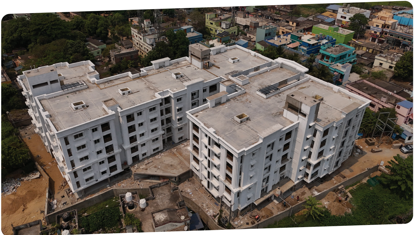
Current stage of Construction
