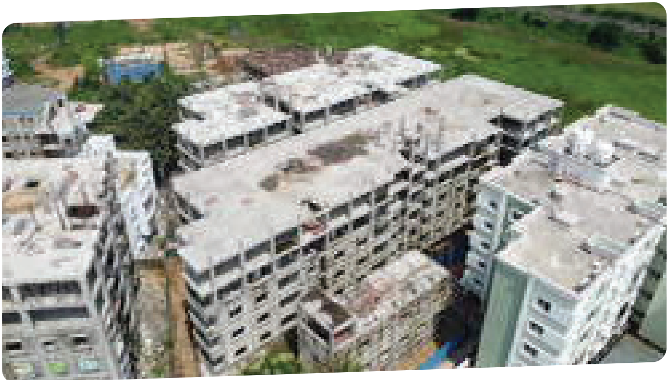
Current stage of Construction
