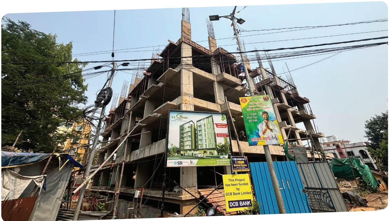
Current stage of Construction
