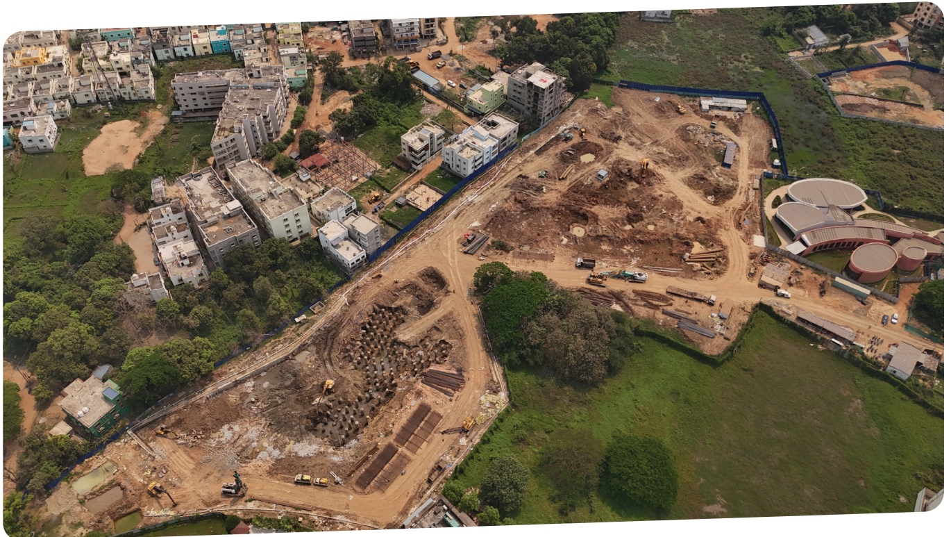
Current stage of Construction
