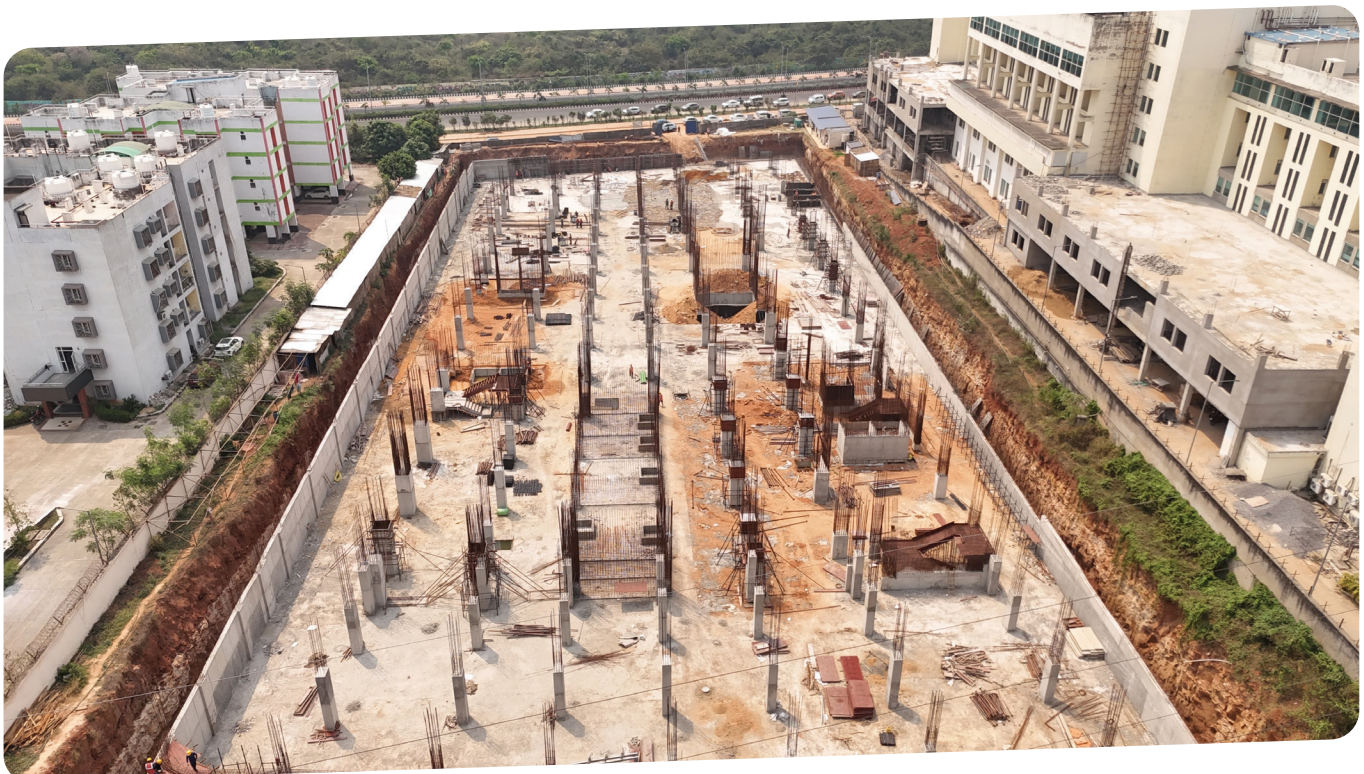
Current stage of Construction
