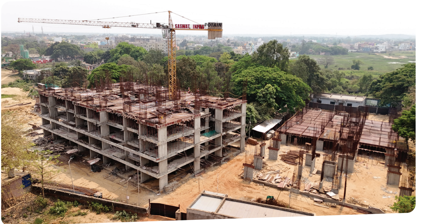
Current stage of Construction
