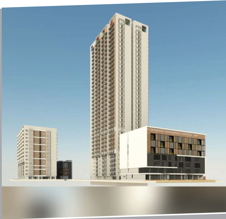
Skycity Towers Patia | Developers : Stalwart Projects Pvt. Ltd B1+B2+B3, G+35 | Area : 10,90,208 Sqft
