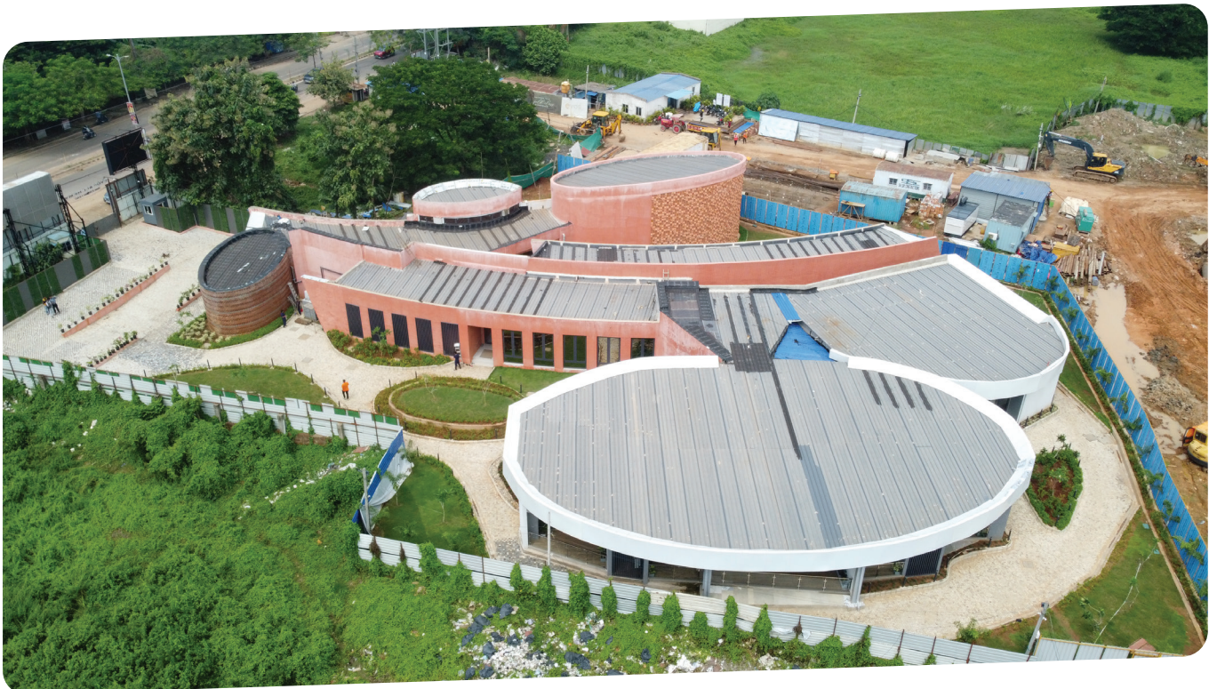
Current stage of Construction
