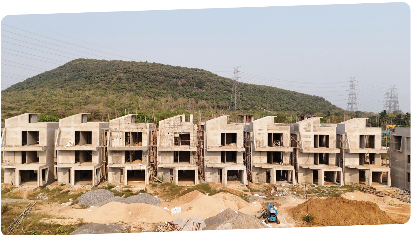
Current stage of Construction
