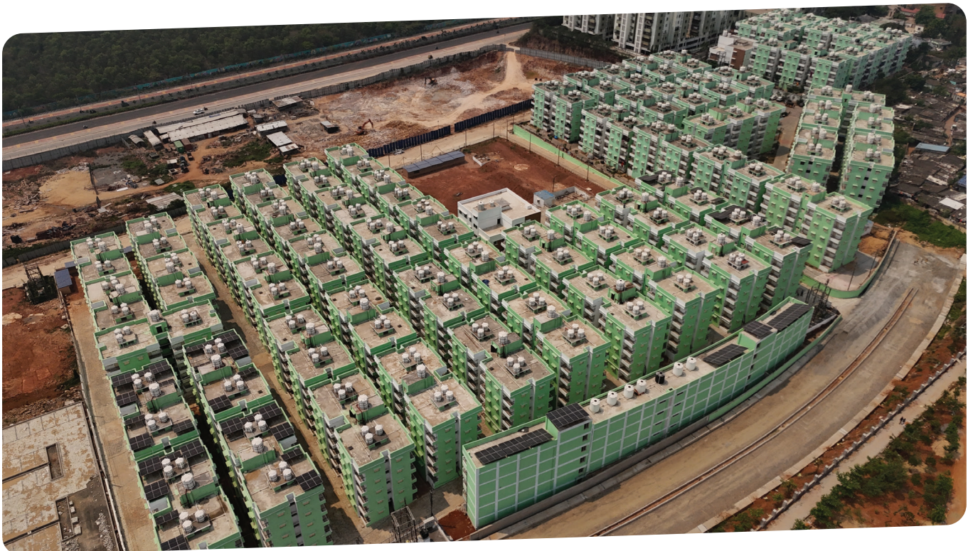
Current stage of Construction
