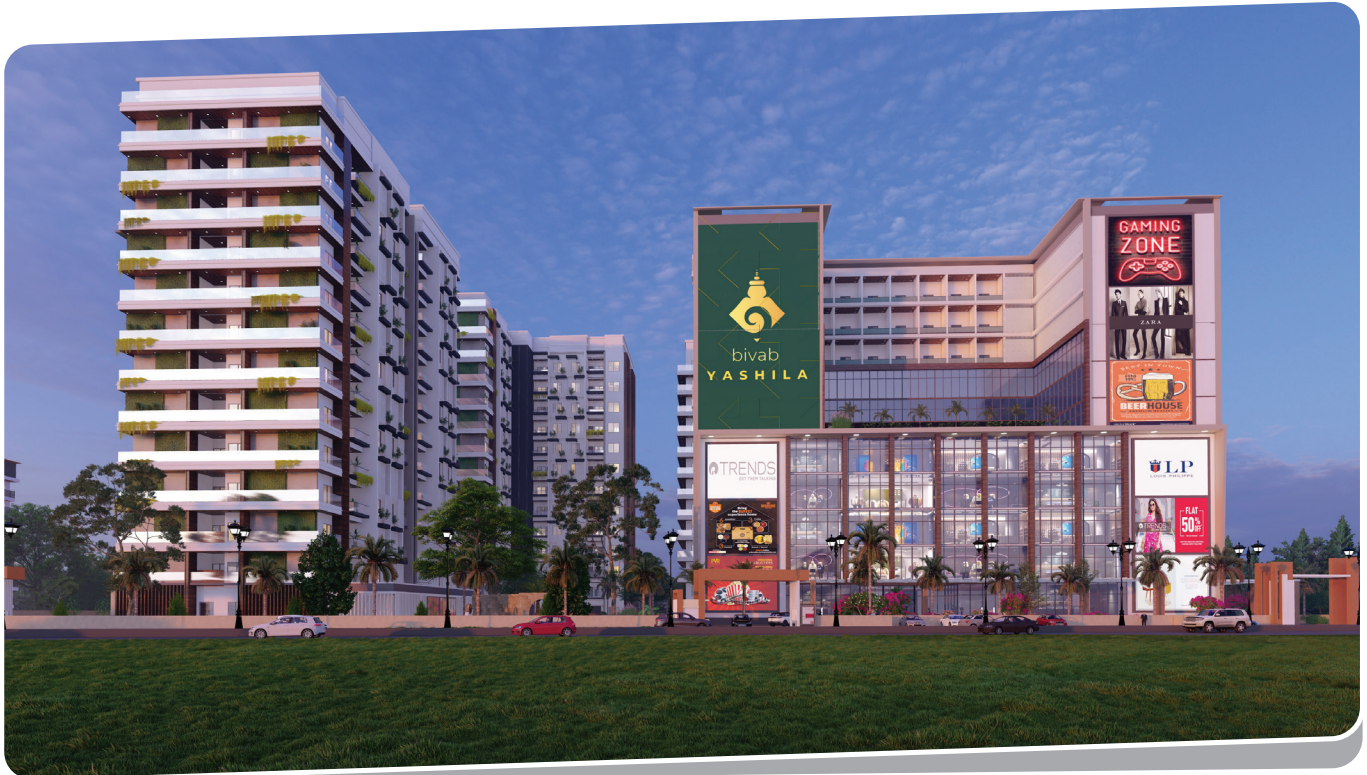
Bivab Yashila, Sipasarubali, Puri | Developers : Bivab Developers Pvt. Ltd B1+B2+G+11 | Area : 5,90,573 Sqft
