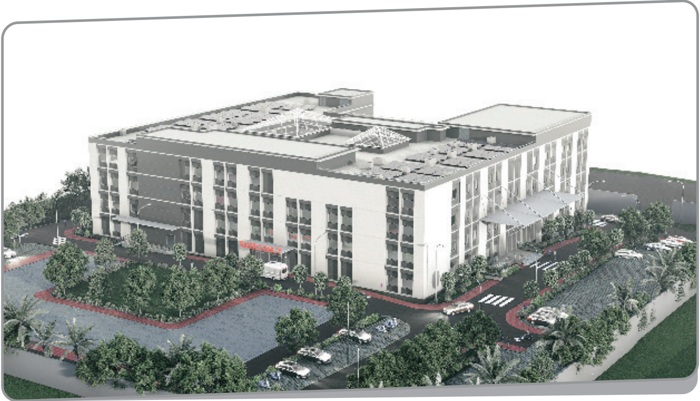
Silicon Hospital, Sambalpur | Developers : CASA Infratech Pvt Ltd B+G+3 floor | Area : 50,000 Sqft
