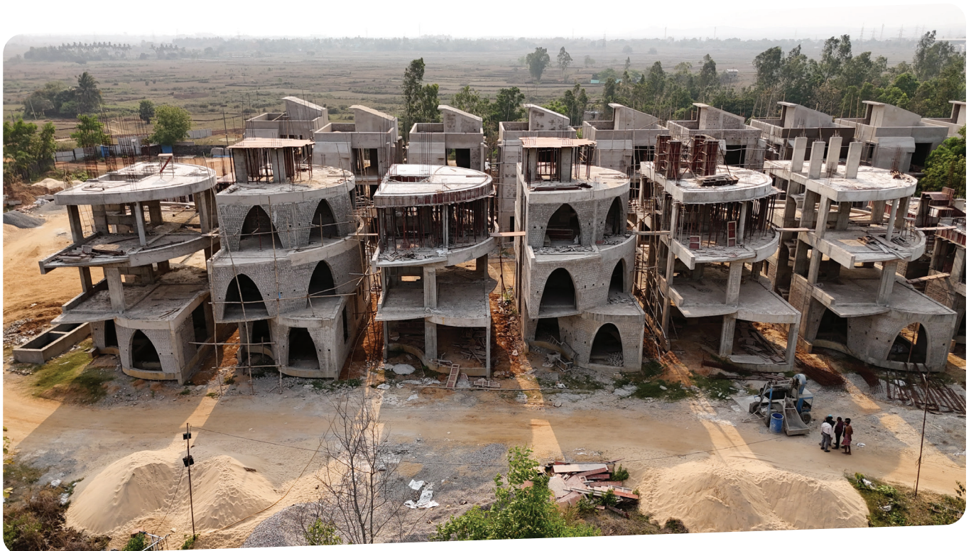
Current stage of Construction
