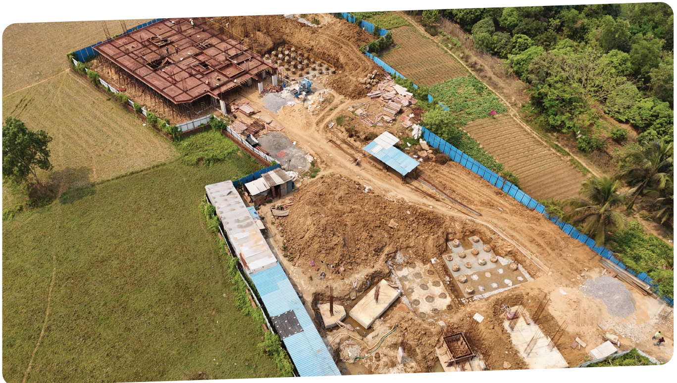
Current stage of Construction
