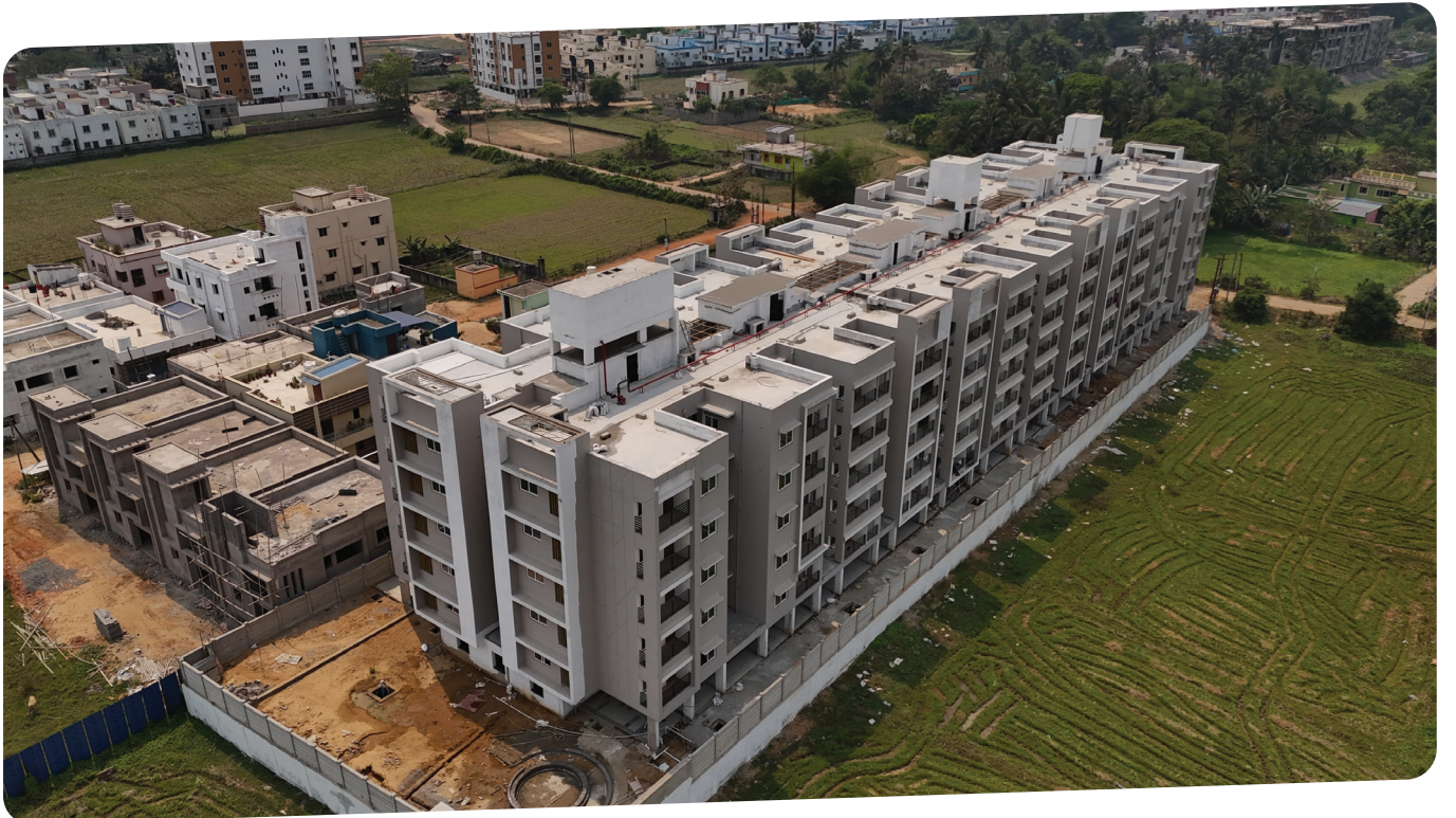
Current stage of Construction
