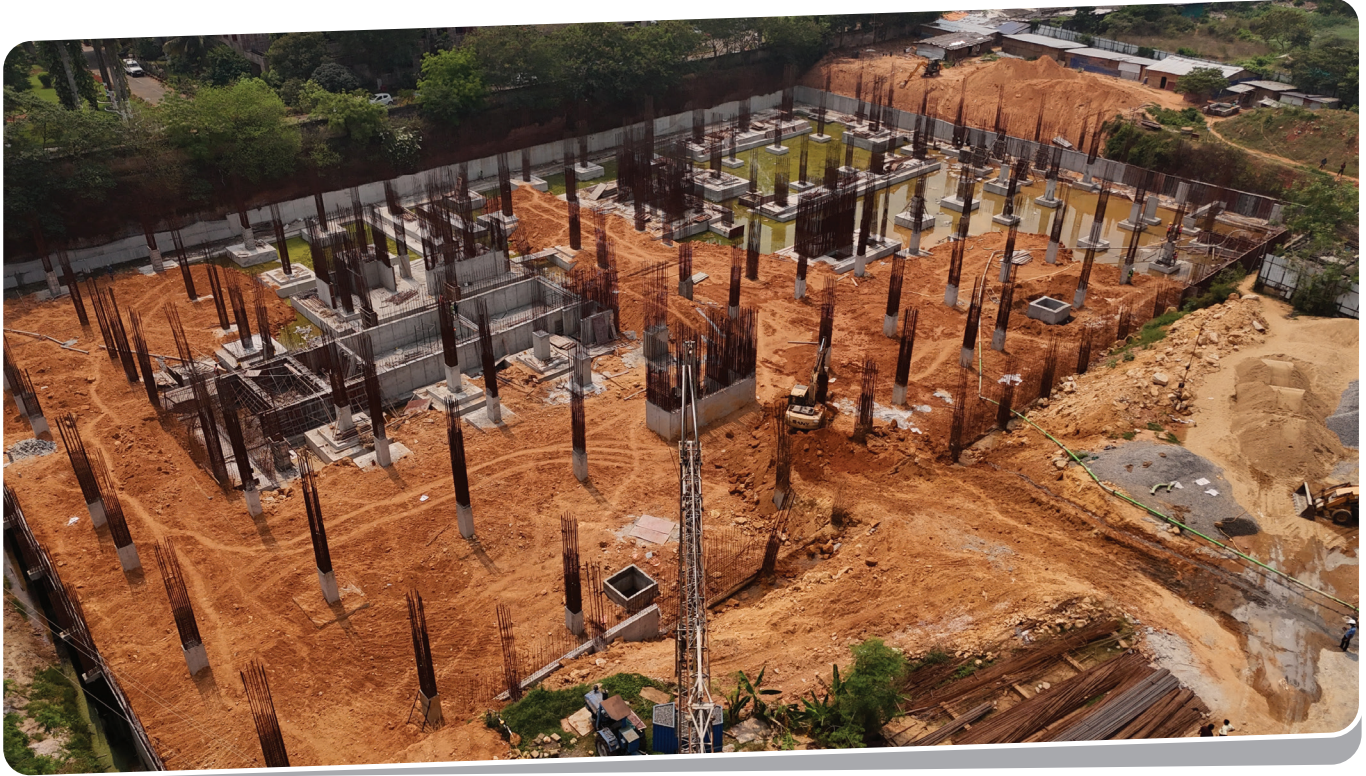
Swami Resorts | Developers : Bhawani Construction Pvt Ltd 2b+G+7 | Area : 6,00,000 Sqft
