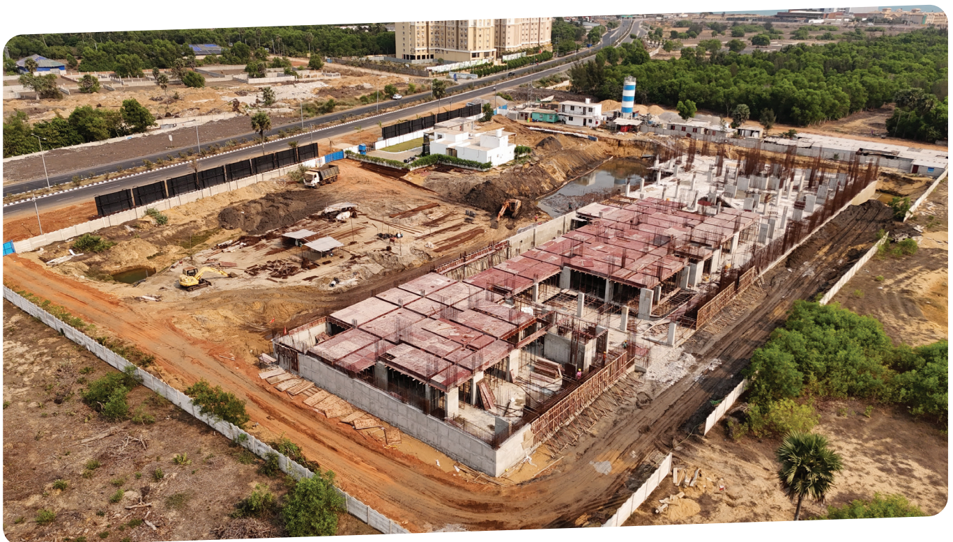
Current stage of Construction
