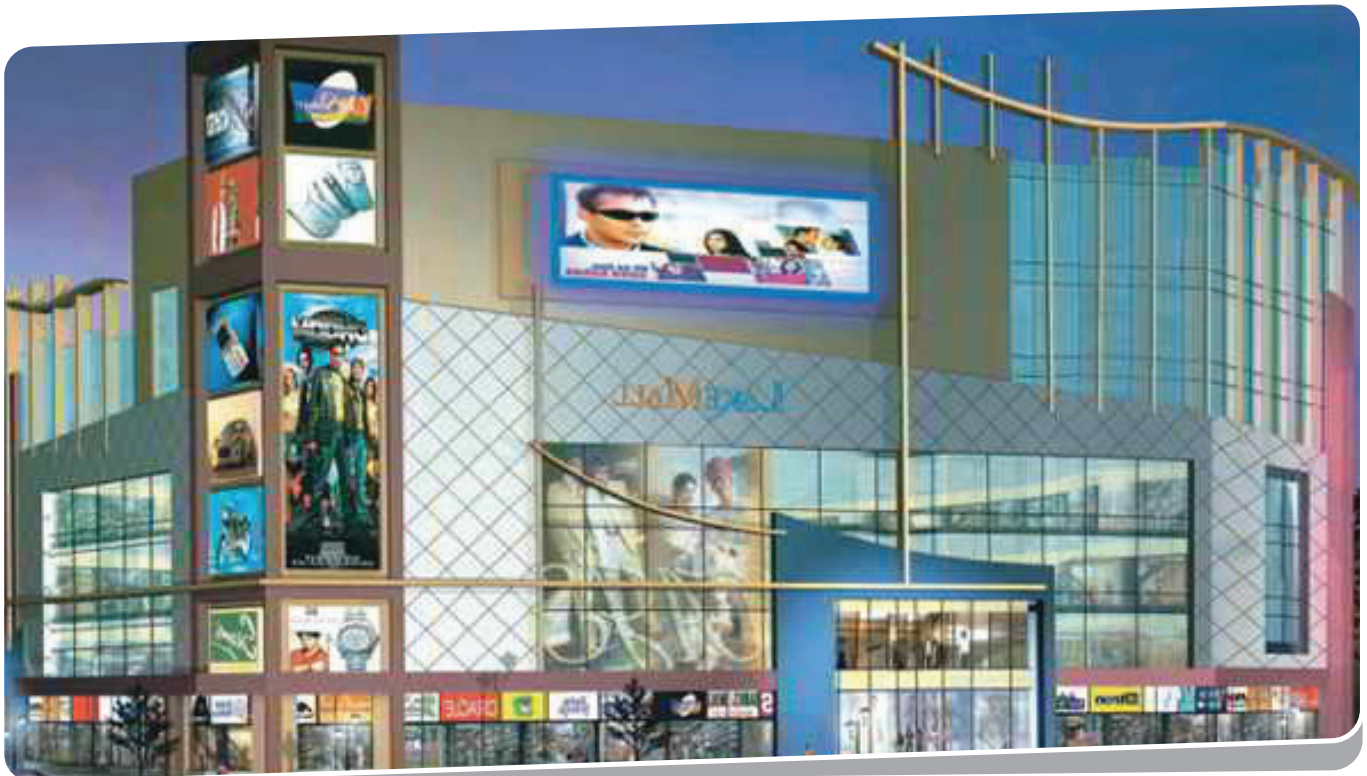
Lake Mall Kolkata | Developers : Venkatesh Foundation Commercial Complex B+G+7 | Area : 1,60,000 Sqft
