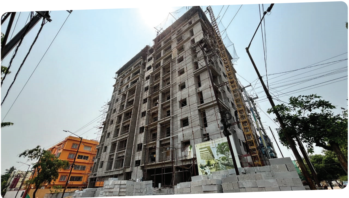
Current stage of Construction
