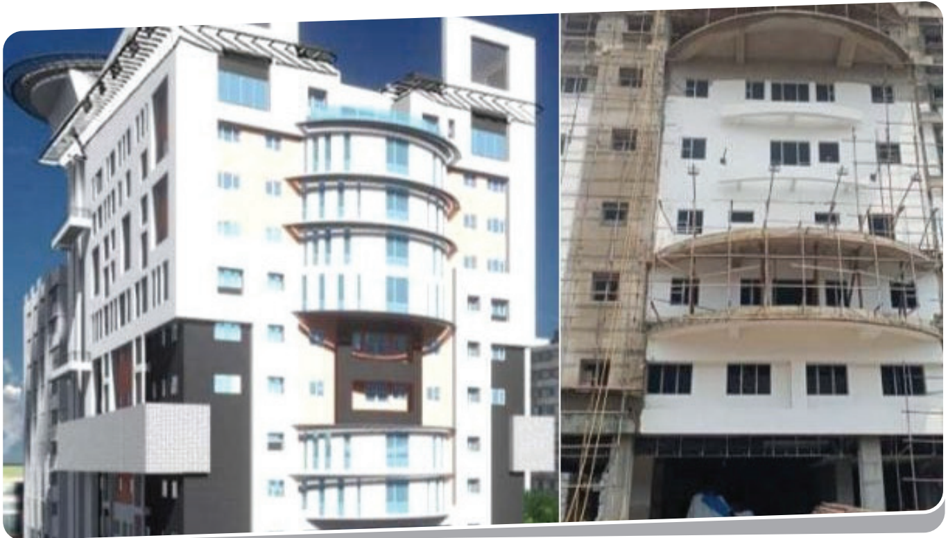
Desun Hospital & Heart Institute Kolkata | Developers : P.n. Memorial Neuro Centre & Research Institute Ltd 2 B+G+10 Storied Hospital Building | Area : 2,07,000 Sqft
