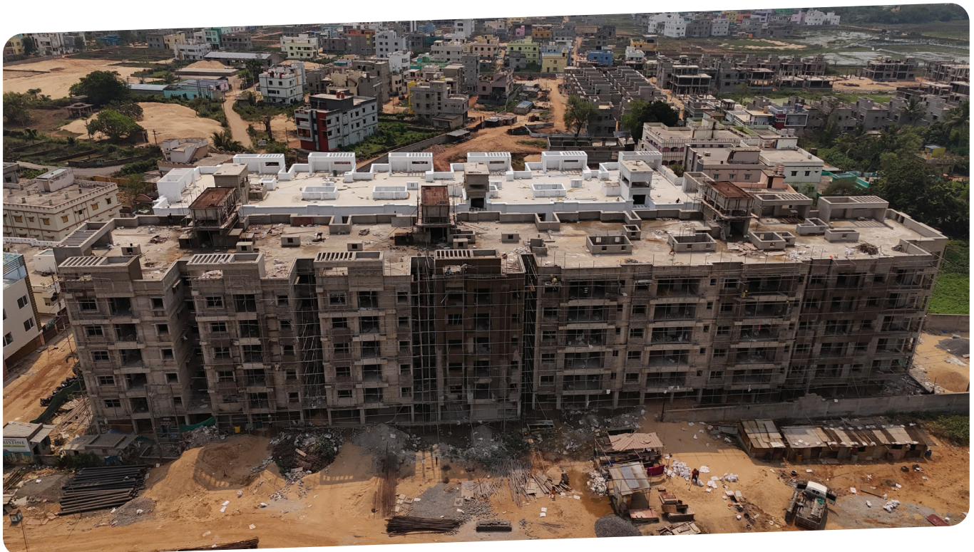
Current stage of Construction
