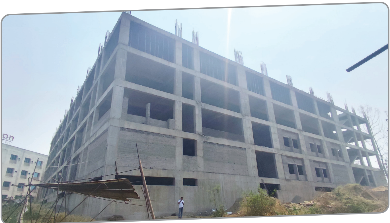
Current stage of Construction
