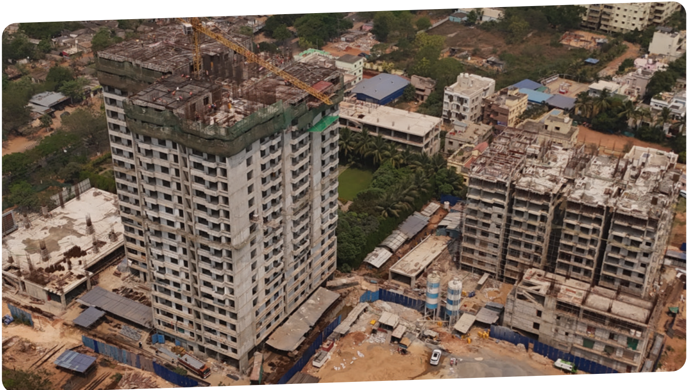
Current stage of Construction
